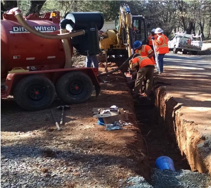
Work on the First Phase of the Hillsdale Project in 2015.
