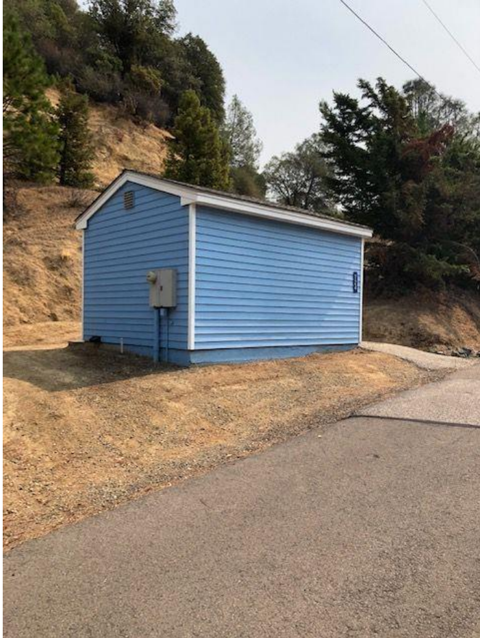
District pump station
