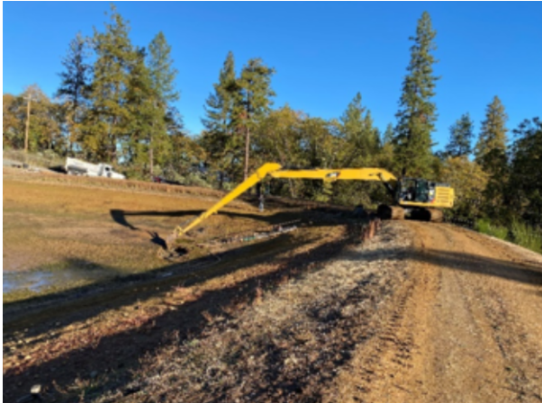
Excavator with 70-foot reach removing sediment from the District's reservoir
